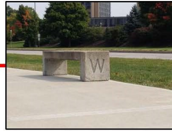
Concrete Benches at ~21' o.c.
