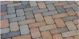
WATER PERMEABLE PAVING
