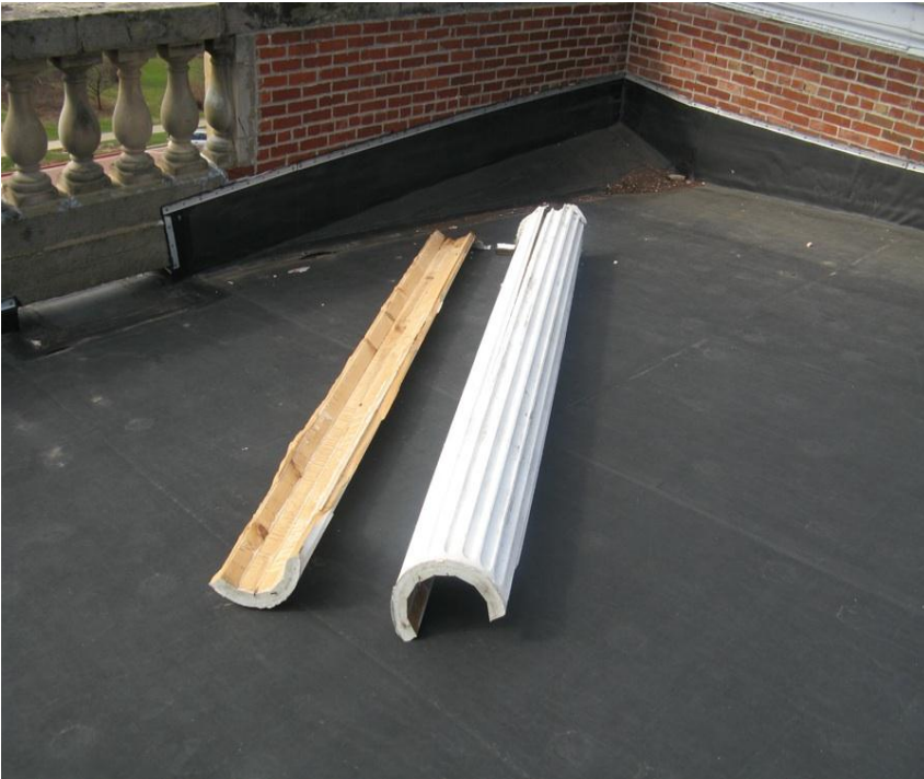
Column on Cupola
