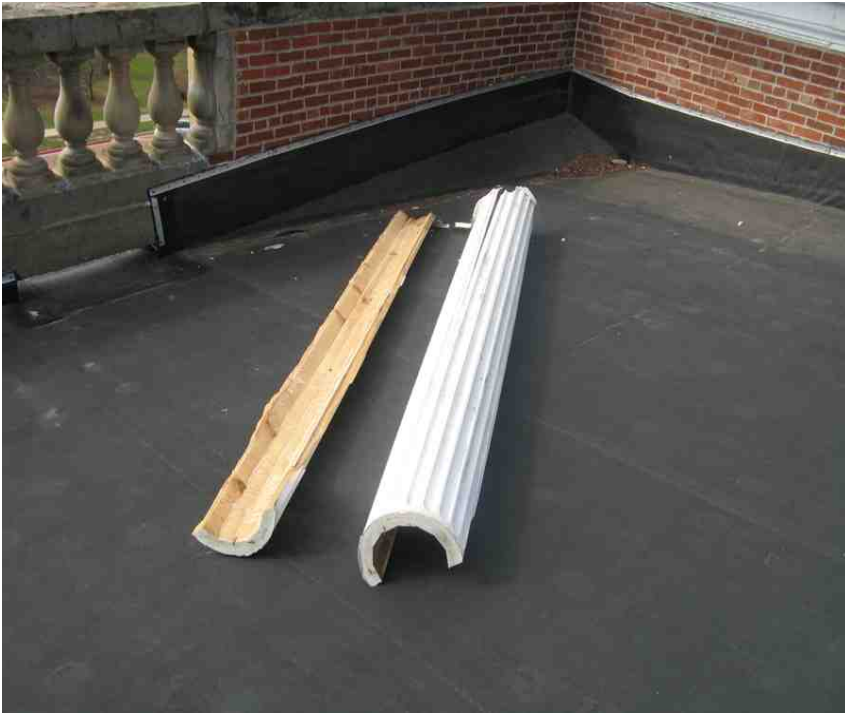
Column on Cupola
